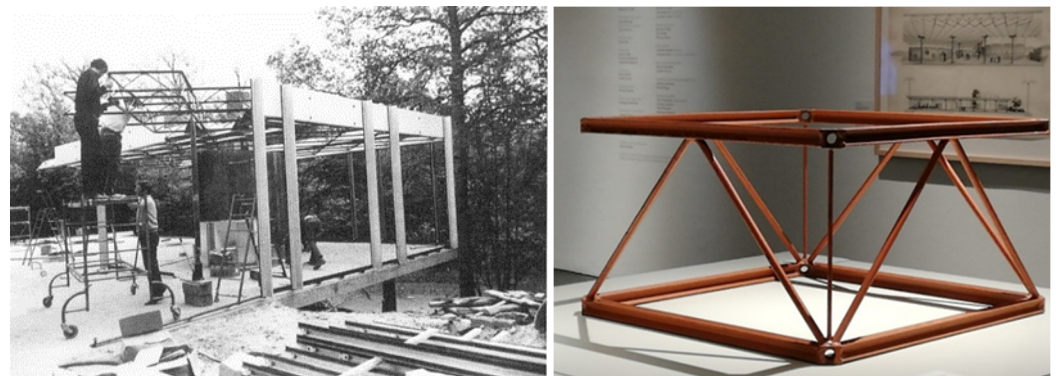
Figure 5. Maison para la Mme. Jaoul . Jean-Claude Drouin, architect; Jean Prouvé, consultant engineer; Léon Pétrouff, engineer; Brisard, construction company (1969) [18]. Model of extendible module by Léon Pétrouff. Photography, authors.
