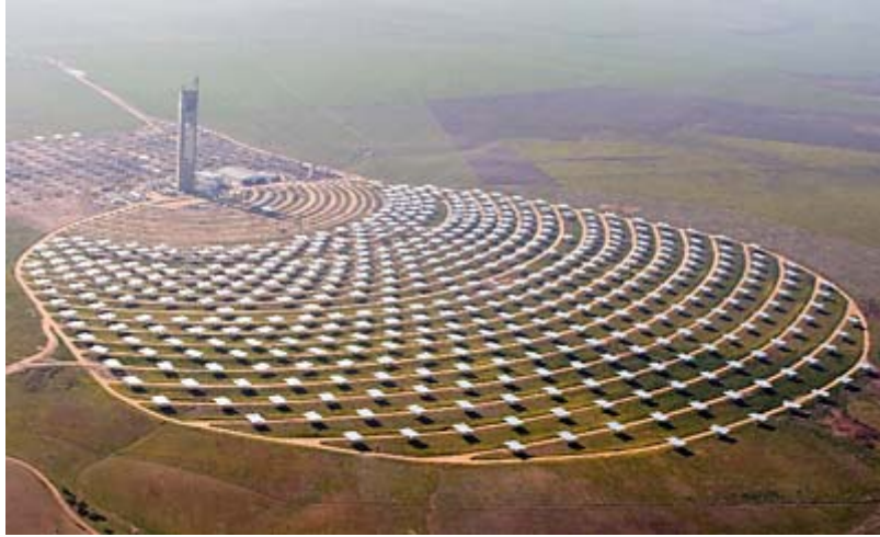
Figure 1. Abengoa Solar plant in Sanlúcar La Mayor [2]
