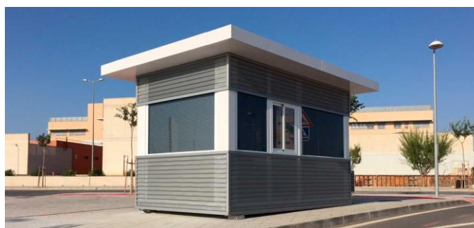
Figura 6.10 Garita de control [34].
