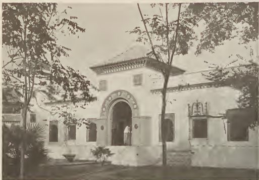
BUILDING OF THE COMPAÑÍA TELEFÓNICA NACIONAL DE ESPAÑA This attractive building will be used for a permanent automatic telephone exchange in Sevilla
