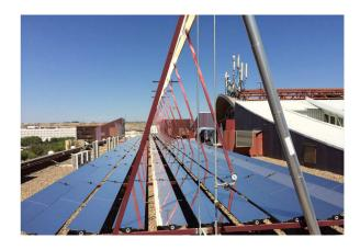
Figure 2: Fresnel collector field
