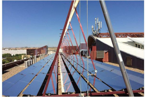
Figure 2: Fresnel collector field
