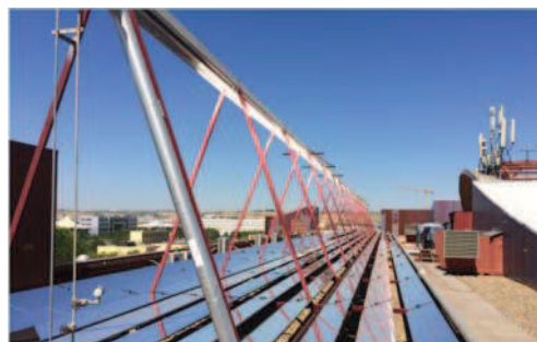
Fig. 3.2. Fresnel collector field.
