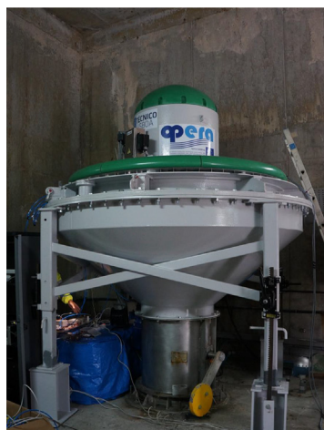
Fig. 12. Biradial turbine during its installation in Mutriku and its characteristic curves and best efficiency point used in CL1.
