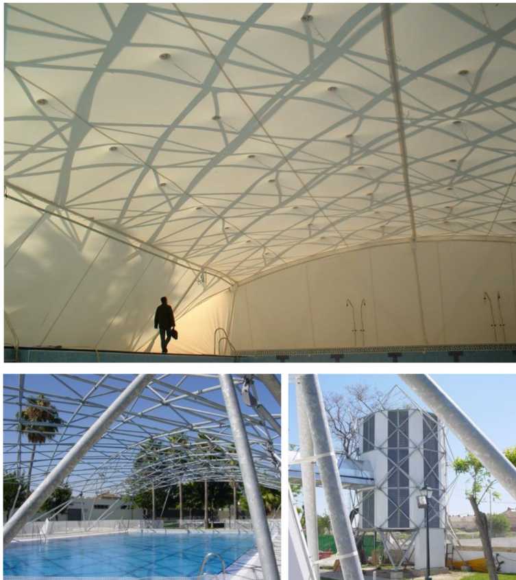
Figure 2: Pool in Gines (Sevilla). Main space and tower's facilities.
