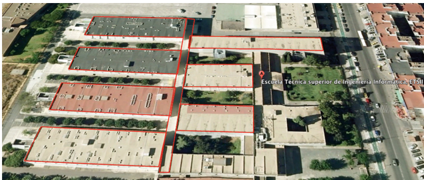
Fig. 2. School of Computer Engineering building
