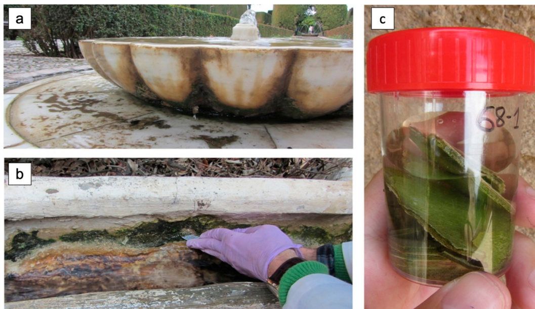
Figure 5. (a) South fountain of the Lower Gardens. The base of the basin, where a dark green mat can be seen, was one of the sampling points; (b) Taking a sample of mineral crust in the Escalera del Agua (Water Stairway); (c) Sample of mineral crust taken in the Washington Irving basin. Photos by G. Alfano.
