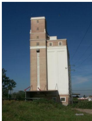
Figure 8: Grain elevator used for the prototype installation.
