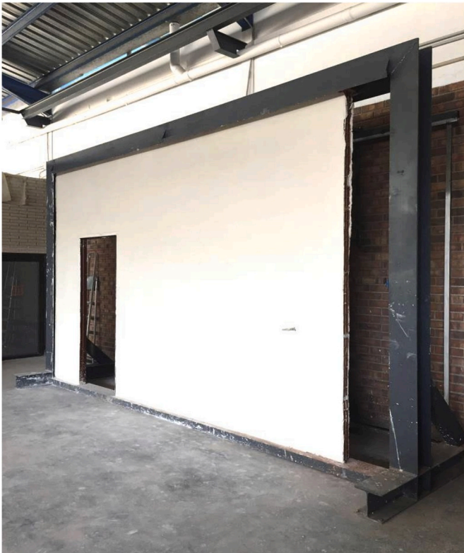
Fig. 6. Image showing the appearance of the prototype wall once finished in the test cell.
