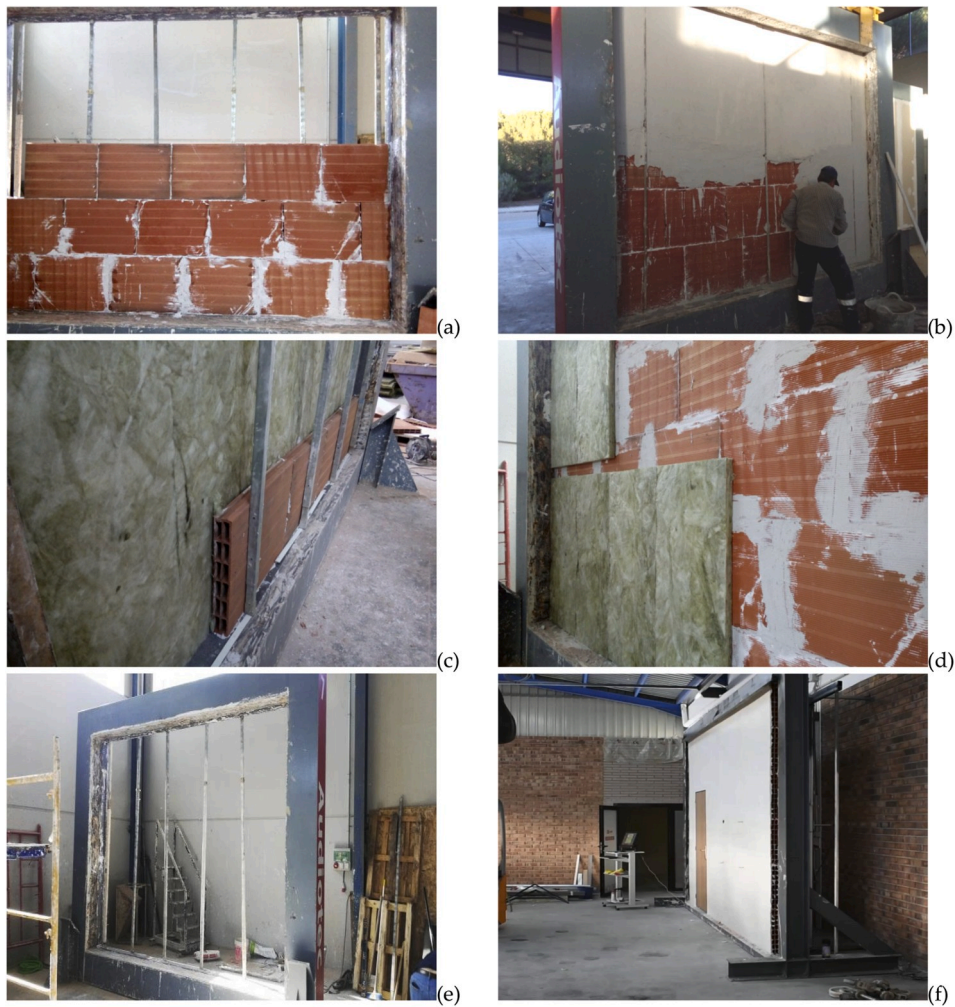
Fig. 16. Assembly process of the tested partitions. (a) Single-sheet partition assembly process, (b) single-sheet partition plaster coating application (c) and (d) two-sheet partition insulation panel assembly, (e) perimeter frame for testing both partitions and (f) executed partition feature.
