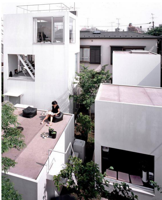
Figura 9. Vista exterior. Casa Moryama. Ryue Nishizawa / SANAA. Ohta-ku. Tokyo, Japan. 2005. https://morewithlessdesign.com/moriyama-house/
