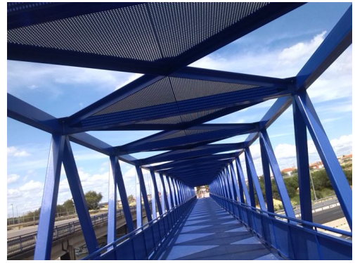
Figure 3. Interior view of the test footbridge
