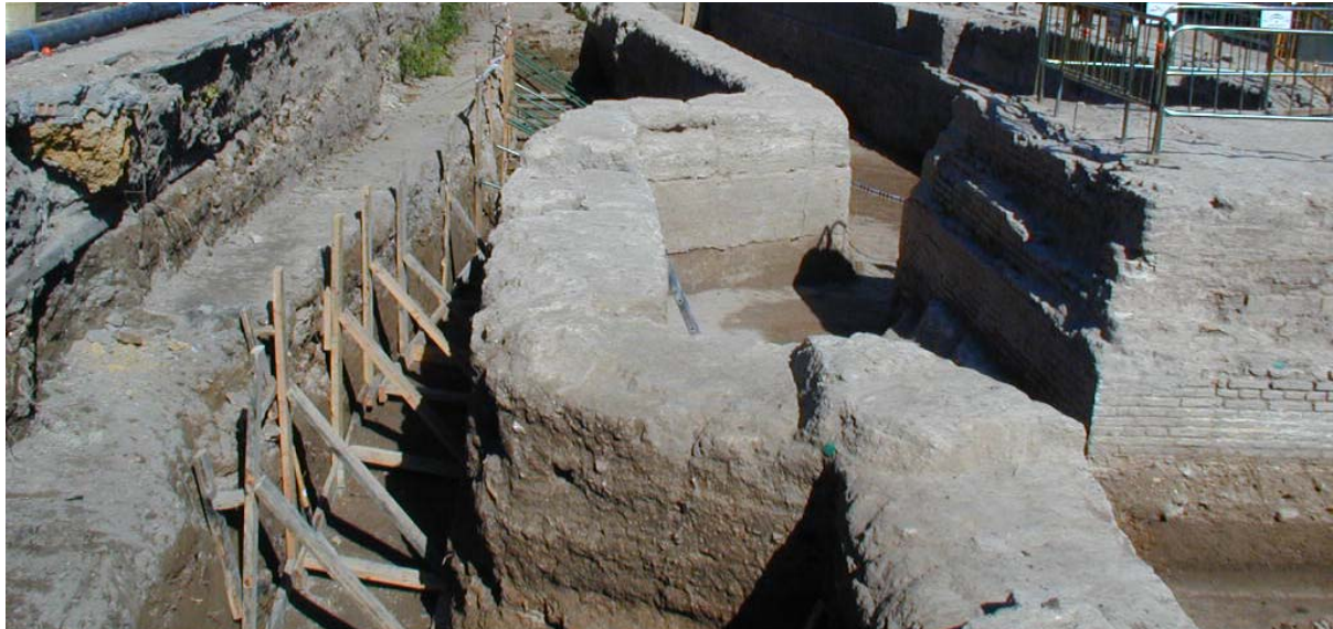
Figure 1. Partial image of the tapial barbican. Photo supplied by the author.
