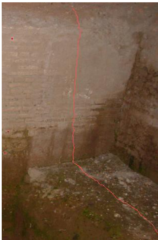
Figure 2: Profile obtained by means a laser plane in a tract of almohade wall in Seville.
