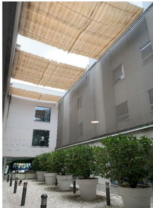
Figure 2. Typical interior courtyard building in Seville. Reference for passive strategies to achieve thermal comfort in hot weather considered in GAUS-D1: Awnings, vegetation, and solar control on facades.
