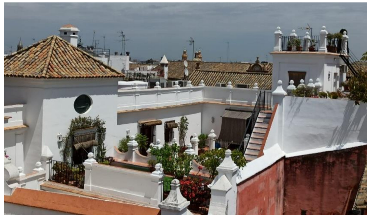
Figure 3. Seville rooftop landscape. Reference for the characterisation of roofs in terms of local construction methods (flat and sloping roofs with Arabic tiles). Source: The authors.
