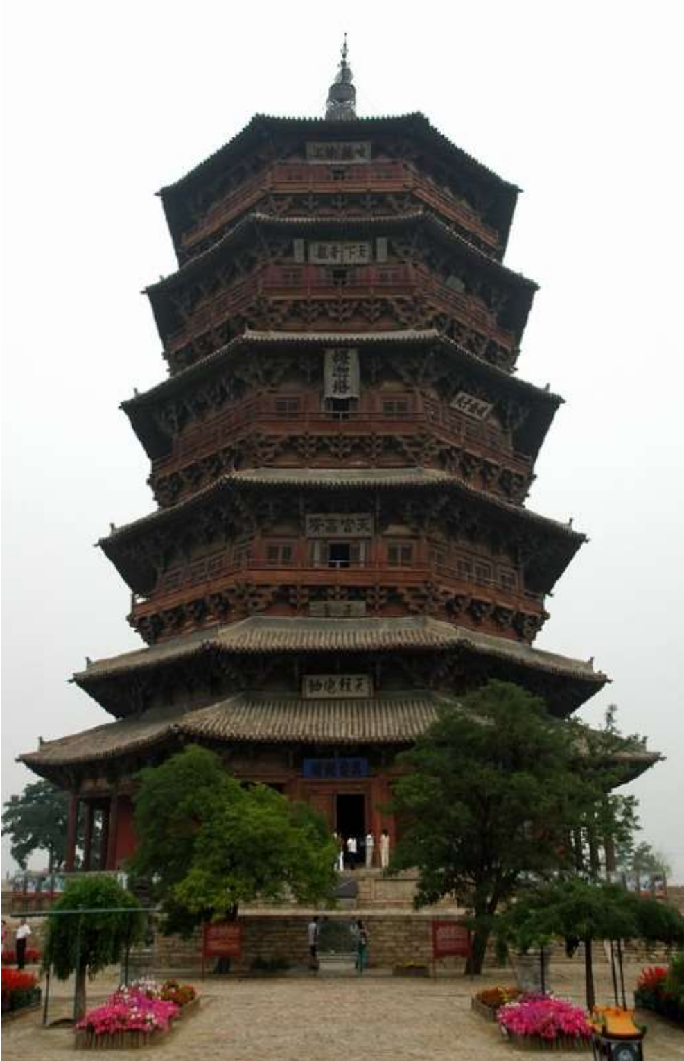
[Figure 110] Seokgatap of Bulgungsa(佛宮寺 釋迦塔) established in 1065, China. Source: Juhjung Lee.
