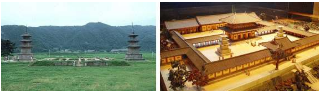
[Figure 196] Front view of Gameunsa Temple and Restoration Mode. Source: Juhyung Lee.
