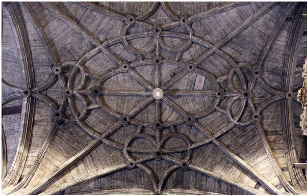
Fig. 13 Second section vault of the church of Santo Tomás in Haro. Photograph courtesy of José Carlos Palacios
