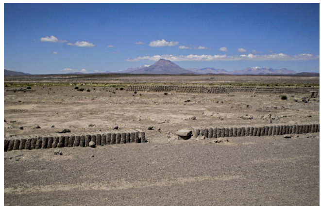
Image 3. ONE STEP IN THE BUILDING PROCESS. After the adobe is formed out of mud and agglutinated thatch, the blocks are piled up and set to dry. Source: Author.
