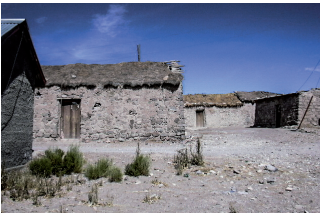
Image 2. APPLIED KNOWLEDGE. Facade built by Thatch-mudded cloth. Stone-walled house. Source: Author.
