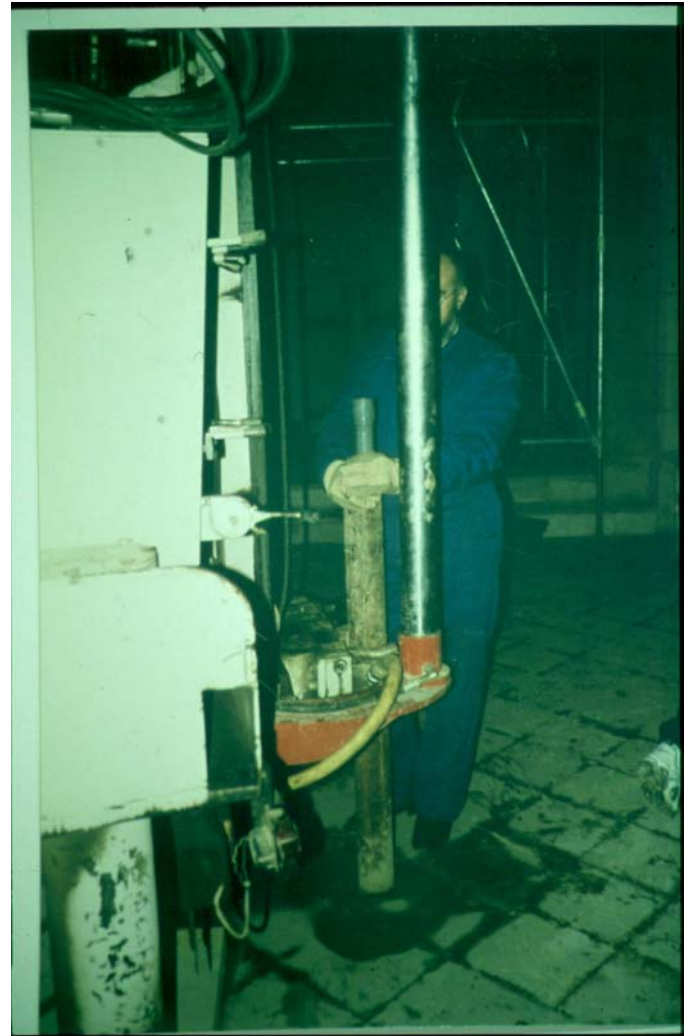
Fig. 2. Bore holes machine working inside the church
