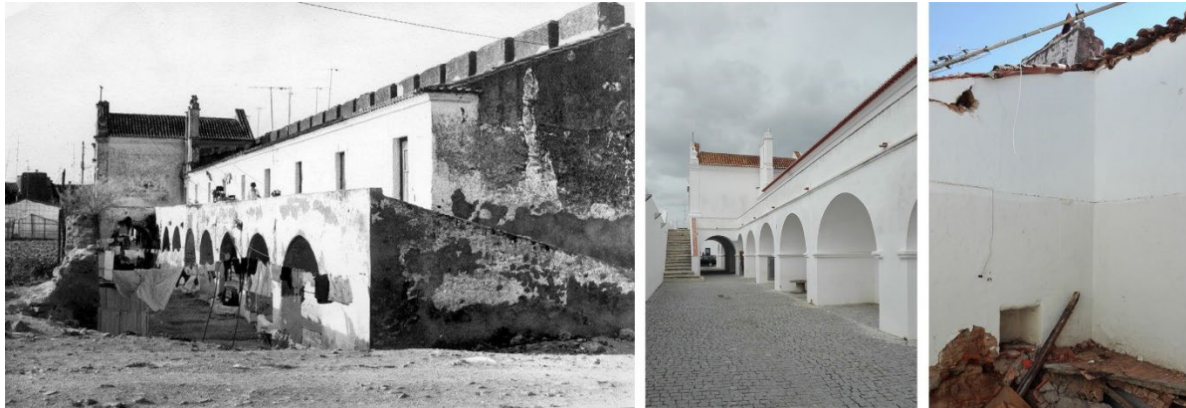
Figure 7. a) Moura's barracks prior to rehabilitation. Source: Diário do Alentejo; b) Moura's barracks after the works; c) ruined module at Estremoz – Rua Direita.
