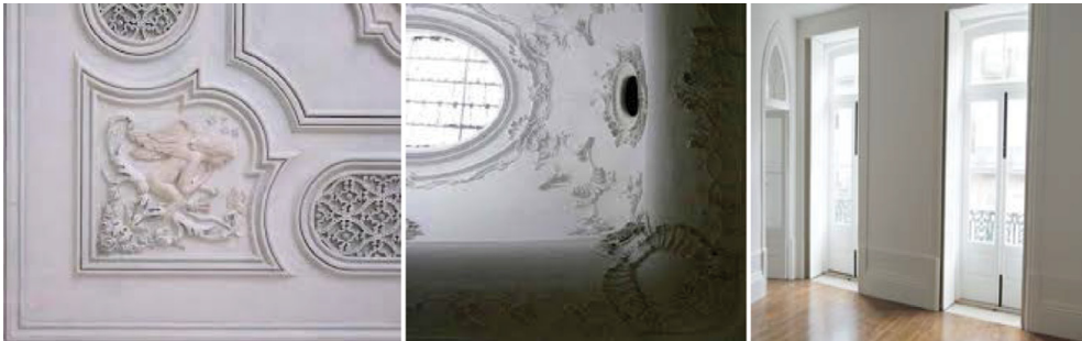
Figure 2: Plaster work (left, middle) and wooden shutters (right).
