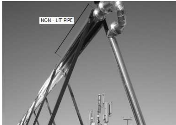
Figure 4. Non – lit pipe due to azimuth.
