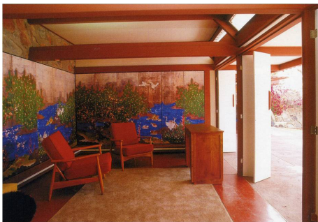
Fig.7. Translucent Panels Used as Light-Shelves, Taliesin West
